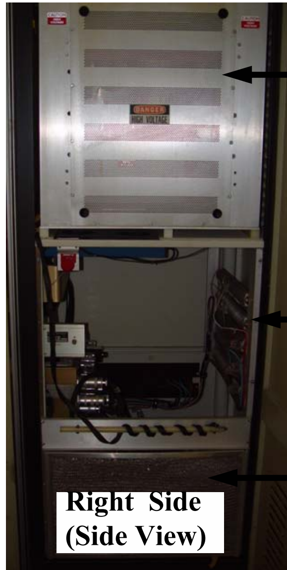
Power Dist. And 4 small Transformers
